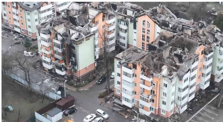
Residential building at 42 Davydchuk Street, Irpin, after occupation. Kyiv region.
