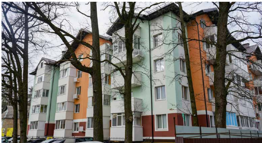
Residential building at 42 Davydchuk Street, Irpin, after restoration. Kyiv region
