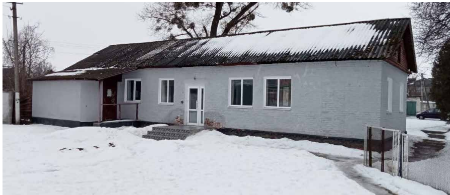
Public restroom in Korop
