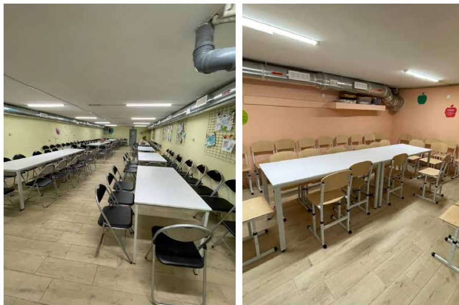
Underground shelter at School No. 58, Mykolaiv 38
