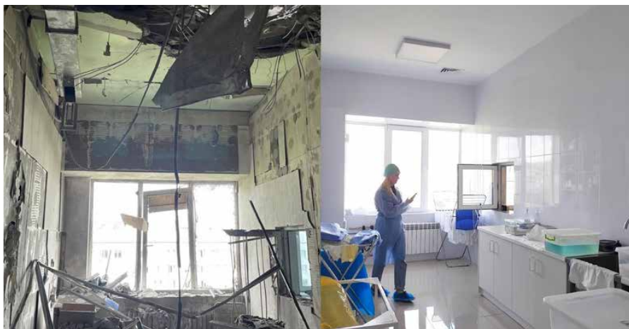
Before and after restoration. Kharkiv Regional Trauma Hospital
