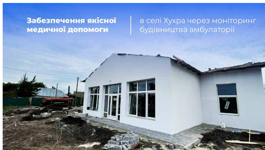
Construction of an outpatient clinic in the village of Khukhra, Chernihiv region 12
