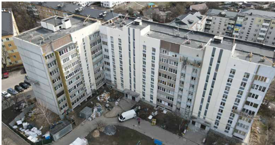
Residential building at 5 Sklozavodska Street in Bucha during the restoration
