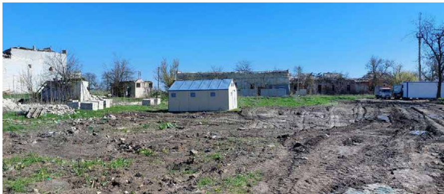
The site where the Security Center is to be built in the village of Posad-Pokrovske. Photo as of May 2025.
