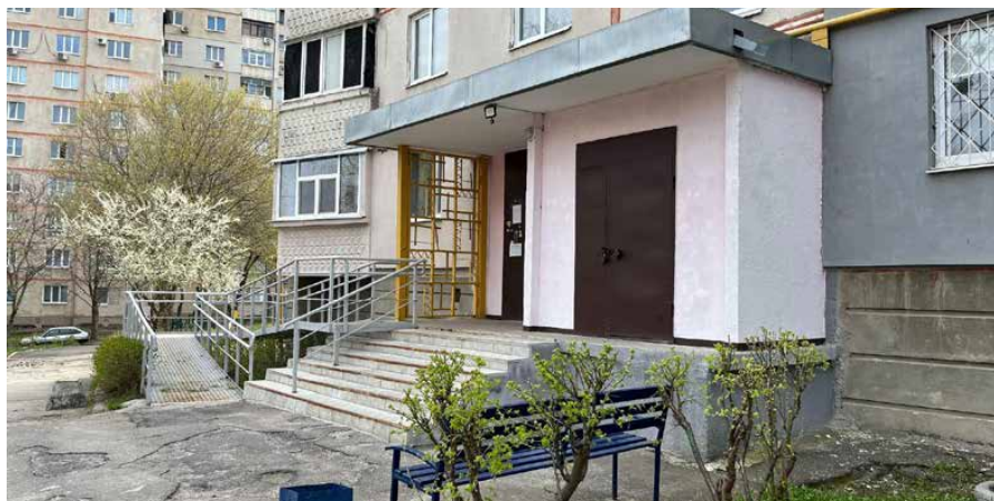
The only entrance in the building at 267 Druzhby Narodiv Street in Kharkiv, where a ramp has been installed.
