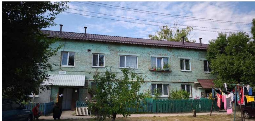
Residential building at 20a Sadova Street, Horenka, Kyiv region, after restoration
