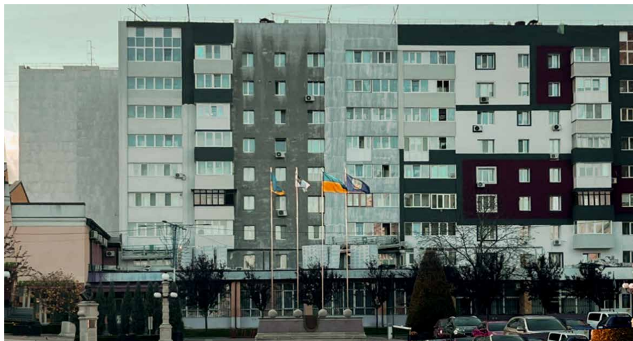
Residential building at 4 Shevchenko Street in Irpin is undergoing restoration. 102
