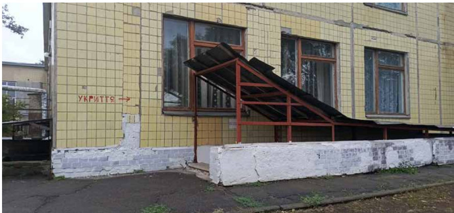
Entrance to the shelter at the Kamianka Gymnasium, Dnipropetrovsk region
