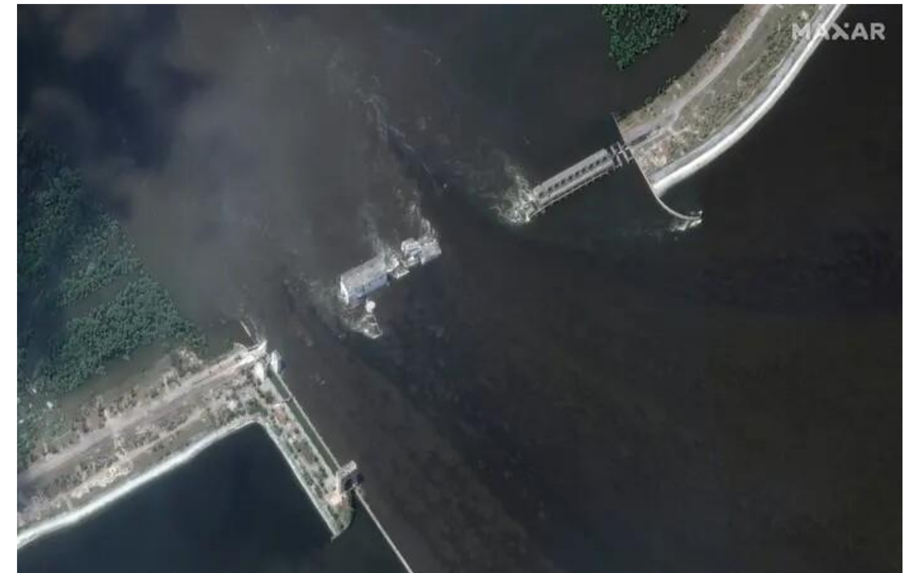
Blown up Kakhovka HPP (6 June 2023)
